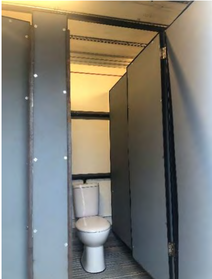
PICTURE – a toilet cubical
