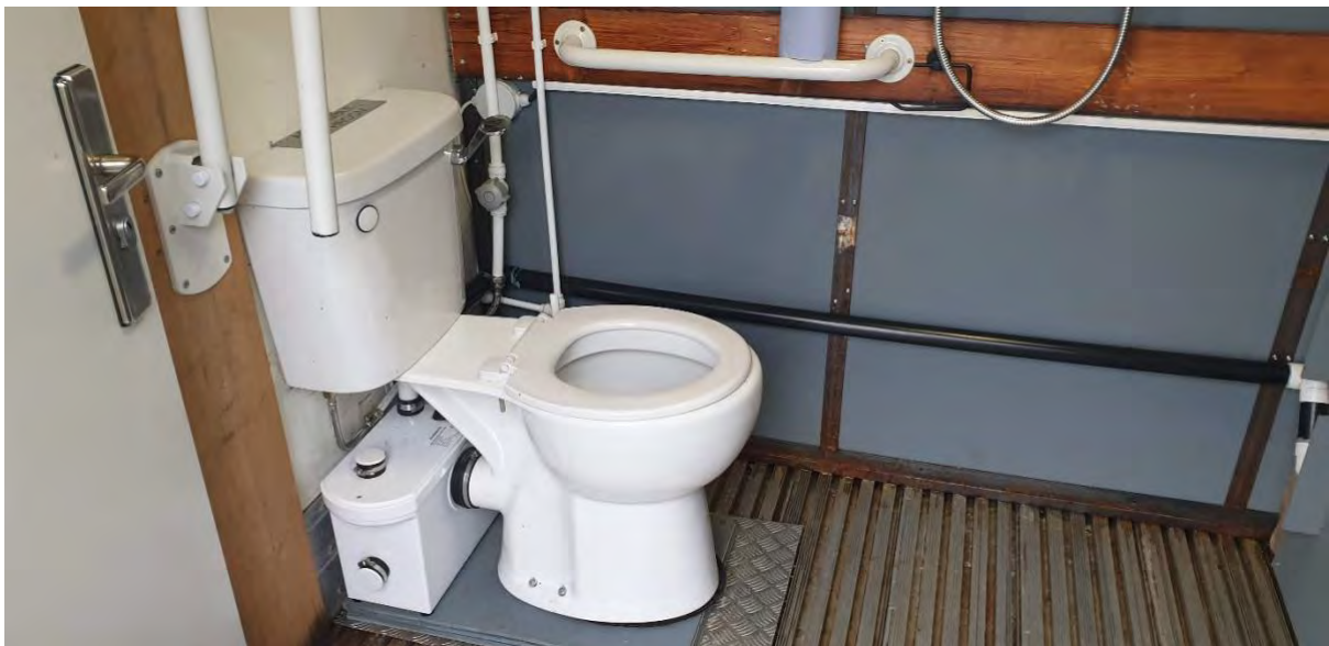
PICTURE – Inside the accessible toilet
