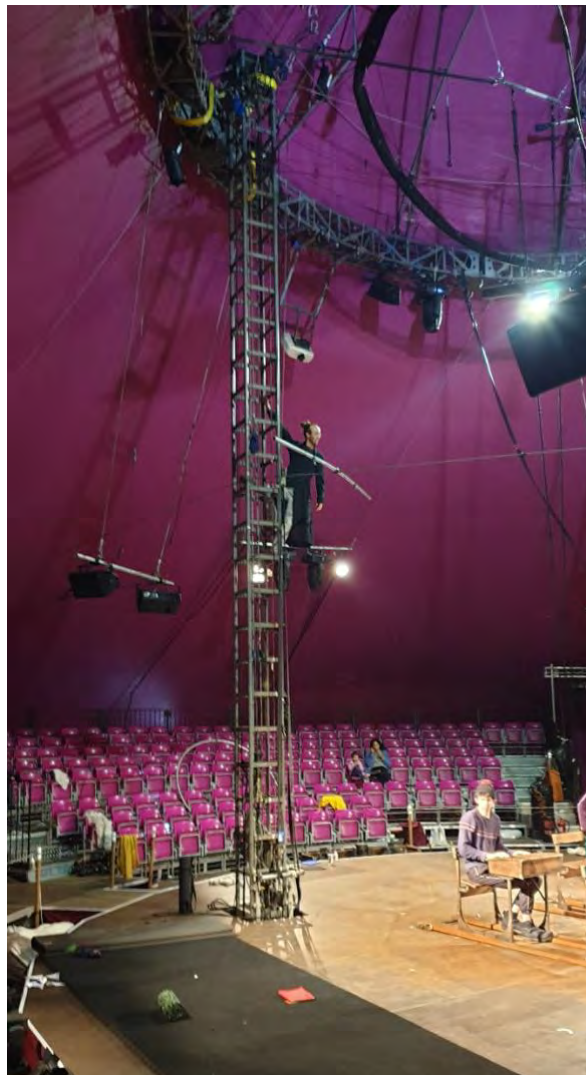
PICTURE – a king pole
